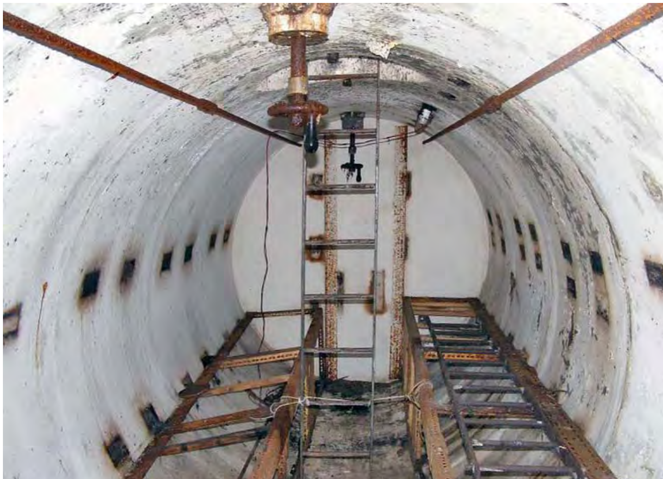
The BX model Fallout Shelter installed by Fall Out Shelters (Deal, Kent) Ltd at Pluckley. The BX is designed to accommodate 12 adults. Photo Mark Russell
